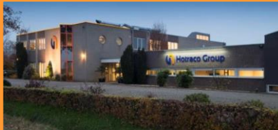
Hotraco HQ & Production
